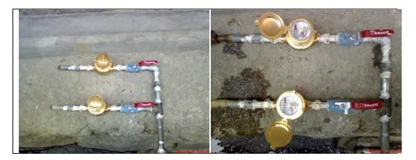
Water meter brand "Kranti Meter" were purchased from Jalandhar, Punjab, and install with each user. For the purpose of control and calculation three meters were also installed at the output of Water Tank Lines.
