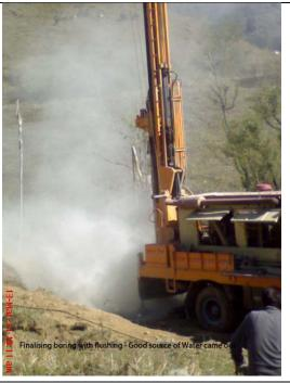
The bore well was fitted with 340 ft. of 2 inches stainless steel top quality GI pipes connected with 12 HP submersible pump on 17<sup>th</sup> March 2011. Three phases electric supply in the name of TCC, Tashi Jong has been taken. The output of submersible pump is connected with the RCC Water tank connected at a distance of about 100 ft. and height of about 40 ft.
